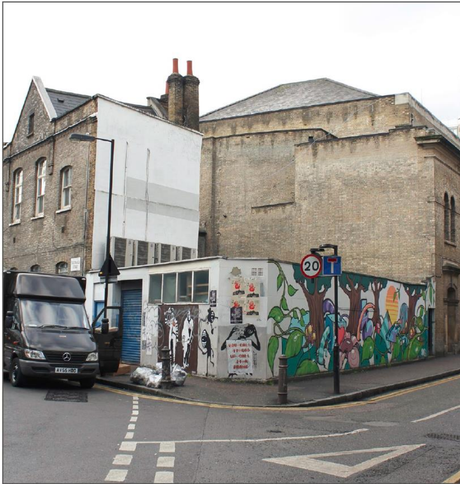
Single storey building at corner of Cowper Street and Tabernacle Street
